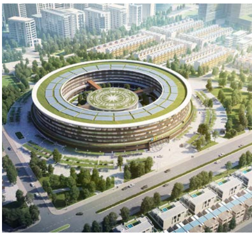
The EDGE-certified FPT Complex in Danang, Vietnam.
